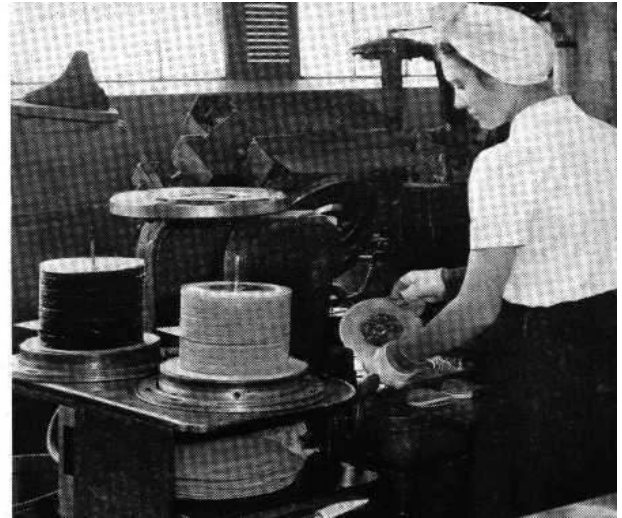
2) 45 rpm record complete with labels is removed from one of the powerful presses at Indianapolis plant
