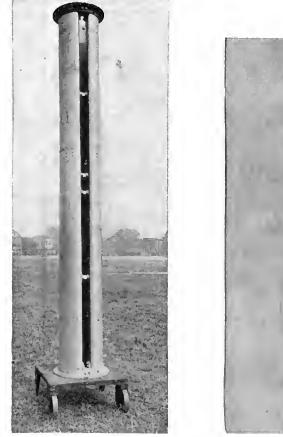
Fig. 1—Single pylon antenna section.
