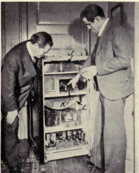
The inside of the Alexanderson television receiver. J points out the neon tube, K the synchronous motor and L the scanning disc. A powerful audio-frequency amplifier of special design is placed in the bottom of the cabinet.
