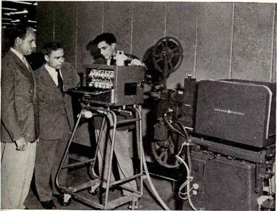
Fig. 4-9. The GE 16 mm film projector is shown in position with the GE film camera on the left. Note that a camera lens is not used.
