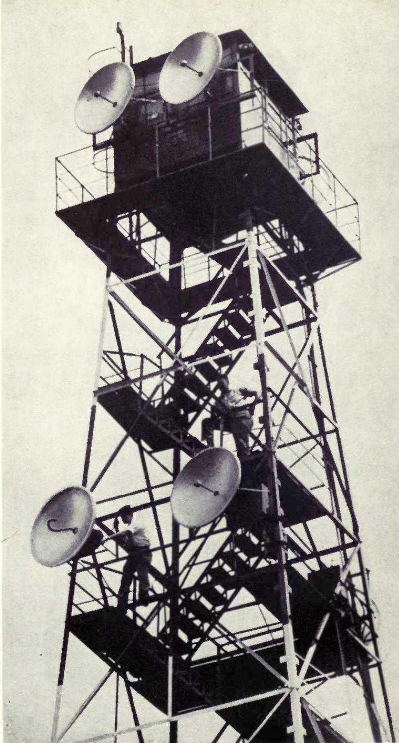
Radio relay stations with 10-foot "dish" reflectors on both sides pick up the television programs and automatically relay them to another relay station or to the main transmitter if it is within range.
