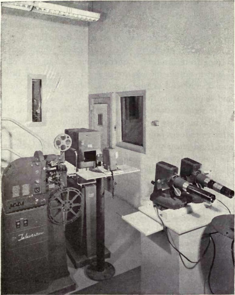
Figure 2-1. Typical film projection room in smaller independent TV station. Space is left on the right of the multiplexer for a second 16 mm projector. The two slide projectors in the right foreground are for station identification and announcements. Station WHIO was constructed by the Austin Company Engineers and Builders, by whose courtesy this illustration appears.
