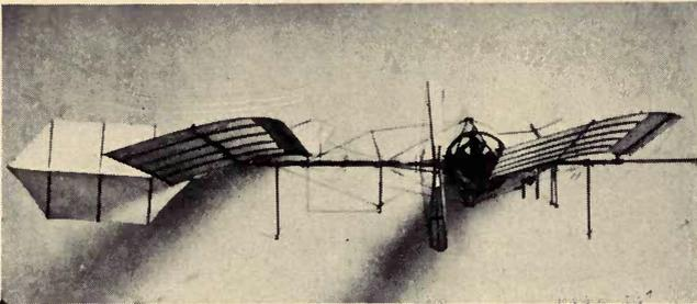
*The Langley tandem monoplane with cambered wings*
