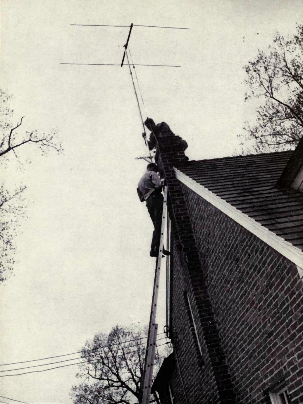
Dipole television antenna with reflector rod.
