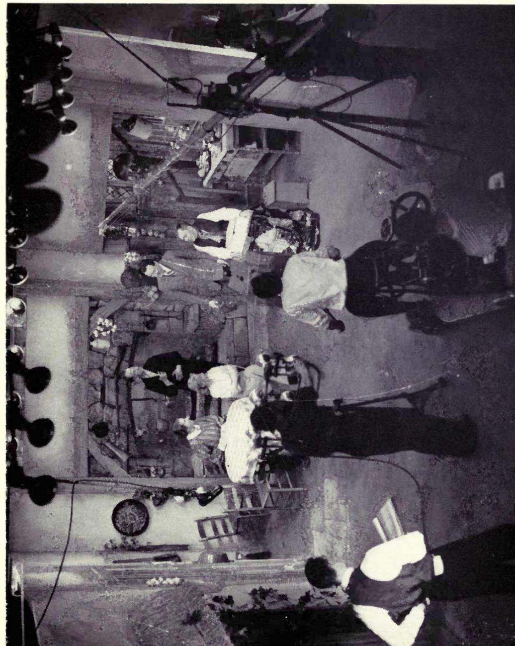
its actors do not stand in a fixed spot and hover around a microphone. The mike must follow the players, so television has adopted the Hollywood technique of hanging the microphone on the end of a long movable boom, out of range of the camera lens.
