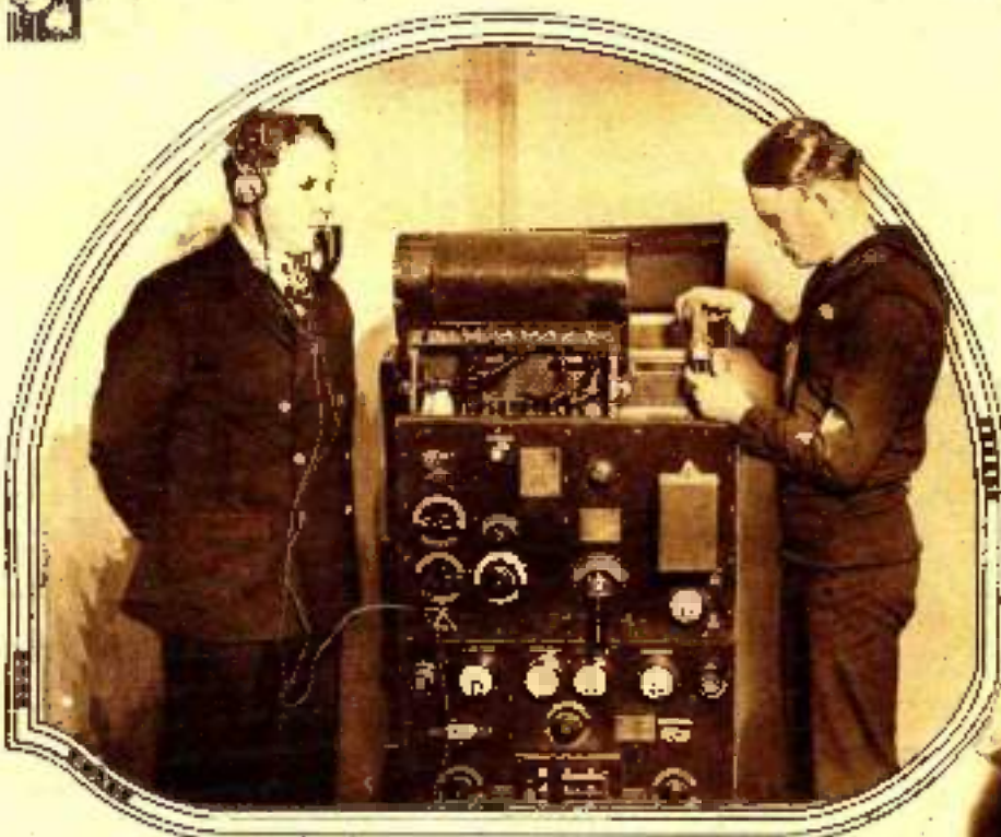
NEW NAVY TRANSMITTER with a power of 200 watts. It employs twelve 50 watt tubes and can be used for C.W., J.C.W. or Radiopneum. It was designed especially for use on the Man o' war. Chief Gunner F. C. Hantz and John Cox are shown demonstrating it at the Radio World's Fair. © Kadel & Harberg.
