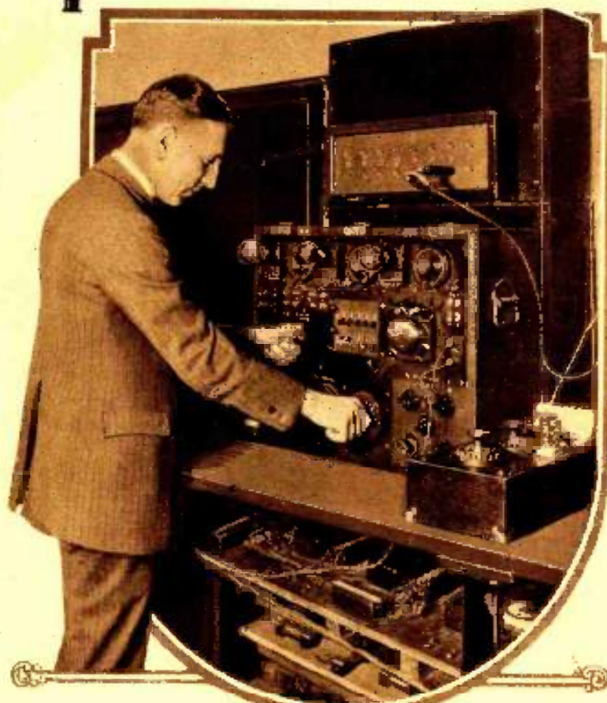
Dr. J. C. Semmler adjusting a vacuum tube amplifier which will produce a pure musical tone of any pitch. Note the various dials under the table.
