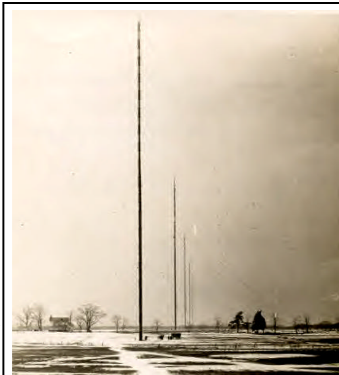
Five of the six 400-foot masts of the Marconi antenna system showing a service team near the base of the closest mast. (Photo courtesy of InfoAge)
