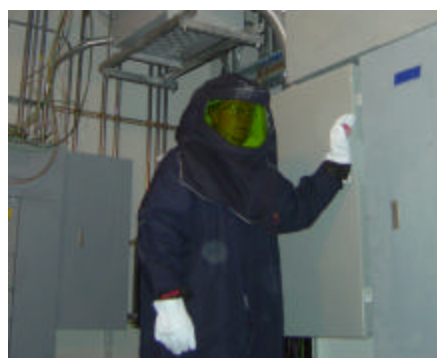
Can he handle the load? Nominee for NJARC president Richard Lee offers this photo in lieu of a candidate's statement. Richard is shown energizing a newly-installed 400 amp, 240 volt, 3-phase service disconnect switch at 1 Bryant Park in New York City.
