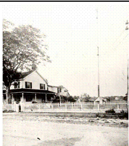
Marconi's 1902 station at Babylon. The house to the left was used as a school and station. The small 12 X 14 foot "radio shack" to the right is what remains today.
