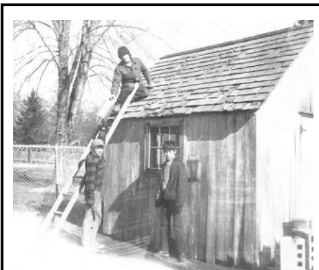
Repairs are performed to a badly deteriorated wireless building prior to its move to the Joseph A. Edgar School.
