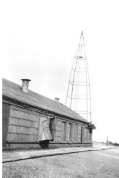
One of the towers on top of the Monument Pottery Co. at 600 Ingram Ave. in Trenton. The tower held up the big, flat top 8-wire antenna of B/C station WOAX which eventually became WTNJ.
