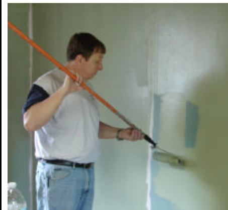
Inside the building. Non-member Ron Beisiada adds the finishing touches.
