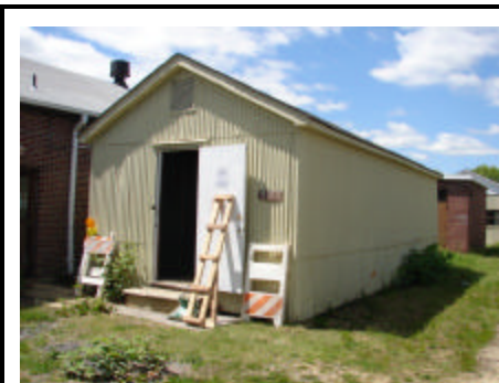
The tube building was originally a support facility for the Camp Evans tube laboratory.
