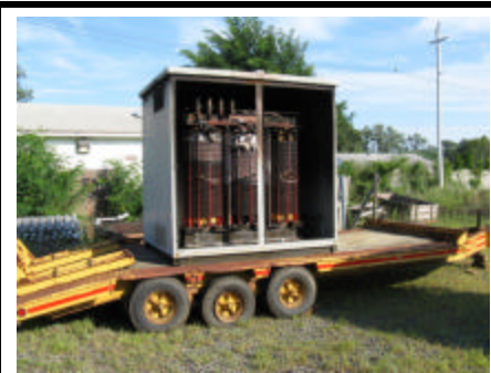
The fire-damaged old transformer on its way out. It was not oil-filled like the new replacement.
