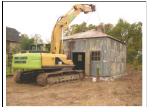
Contractors hired to demolish Brookdale College buildings prepare to move Bldg. 9115 to its new home. Compare this photo to the SCR-271 building at Twin Lights. The amplidyne, fuse panel and control panel were moved to safe storage by Joe Giliberti. Ray Chase is on the prowl for other original components.
