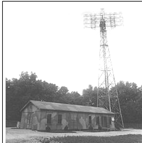
An SCR-271-D radar at the Evans Signal Laboratory with shelter for components and operating personnel. The antenna has been modified for a PPI display.
