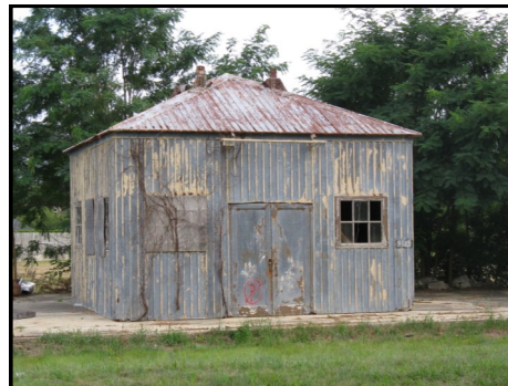
Building 915 at its new location.
