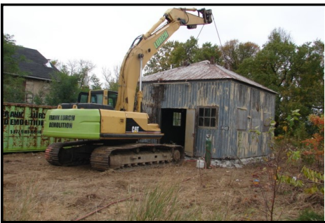
The initial lift had to be abandoned; the demolition company did not appreciate the weight of the building and a special crane had to be brought in.
