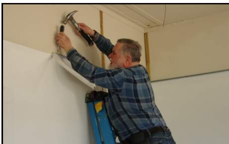
Member Vince Lobosco removes ceiling tile supports in preparation for room repainting and restoration.
