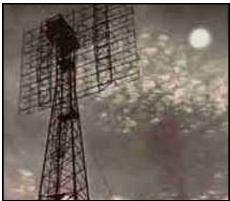
Special radar antenna array of 64 dipoles. It could change azimuth but not elevation.
