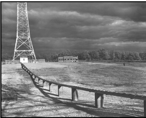
This is a rear view of the WEAJ antenna system, showing the elevated raceway supporting the coaxial transmission line that connected the two towers.
