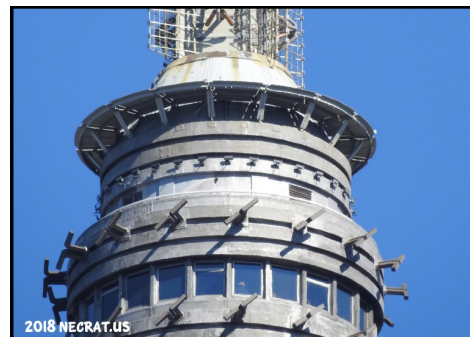
The Alford antenna showing its 32 elements arranged in two rings above and below the observation gallery on the 102nd floor.
