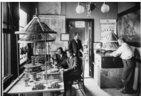
Charles "Doc" Herrold (center, in the doorway) powered his early-1900s San José, Calif. AM radio station with arc technology of his own design. This photo appears to show two of the converters built into the table at the left. A phonograph turntable is visible as is a microphone. Although Federal's transmitters were designed to operate in the
