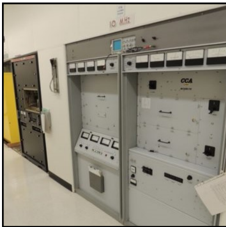
WWV 10 MHz transmitter and standby.
